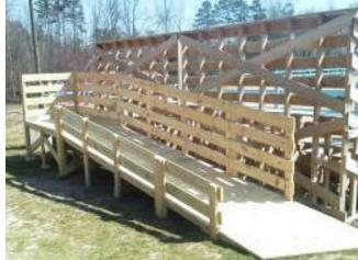
Note: These plans can be used either exactly as drawn or as a guideline for your particular needs. The location where we built our mounting platform had a slight slope to it, so the ramp length ended up being about six feet shorter than what is shown for when level land is available, while retaining the designed ramp angle (see photo). Also, Sally decided that she wanted the safety rail on the mounting side to only be 18" high so that a helper can more easily access the handicapped rider.
